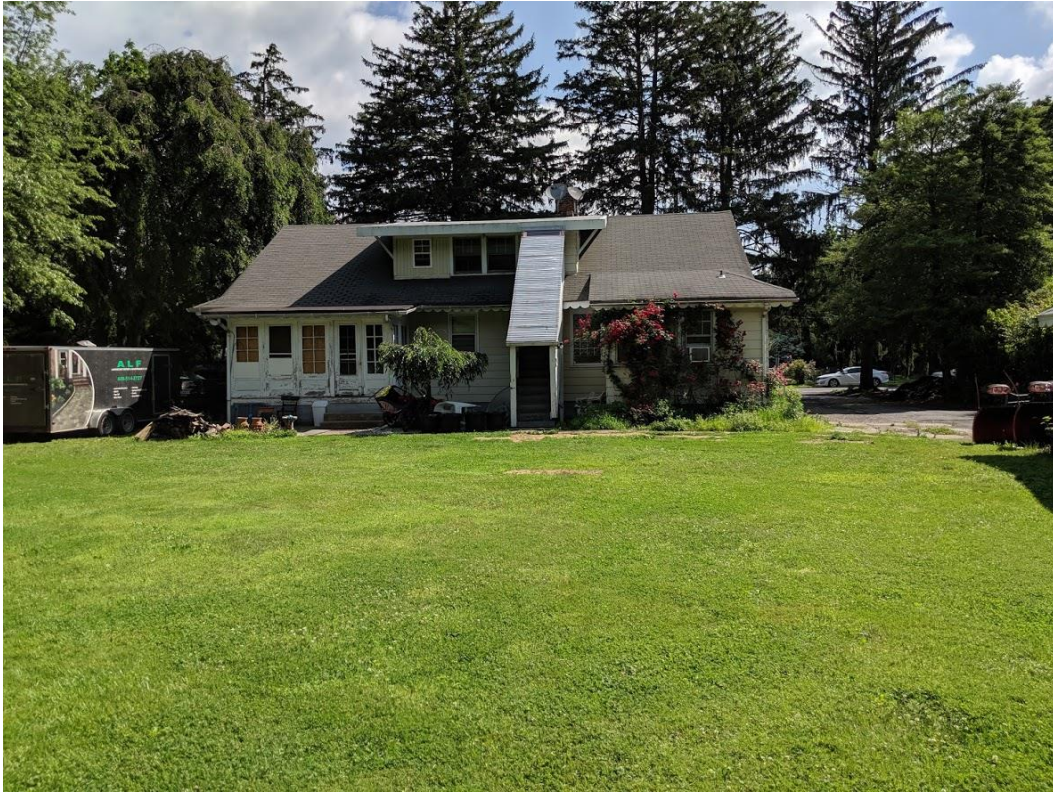
Photograph 42: Block 39 Lot 7 Rear Façade and Rear Yard
