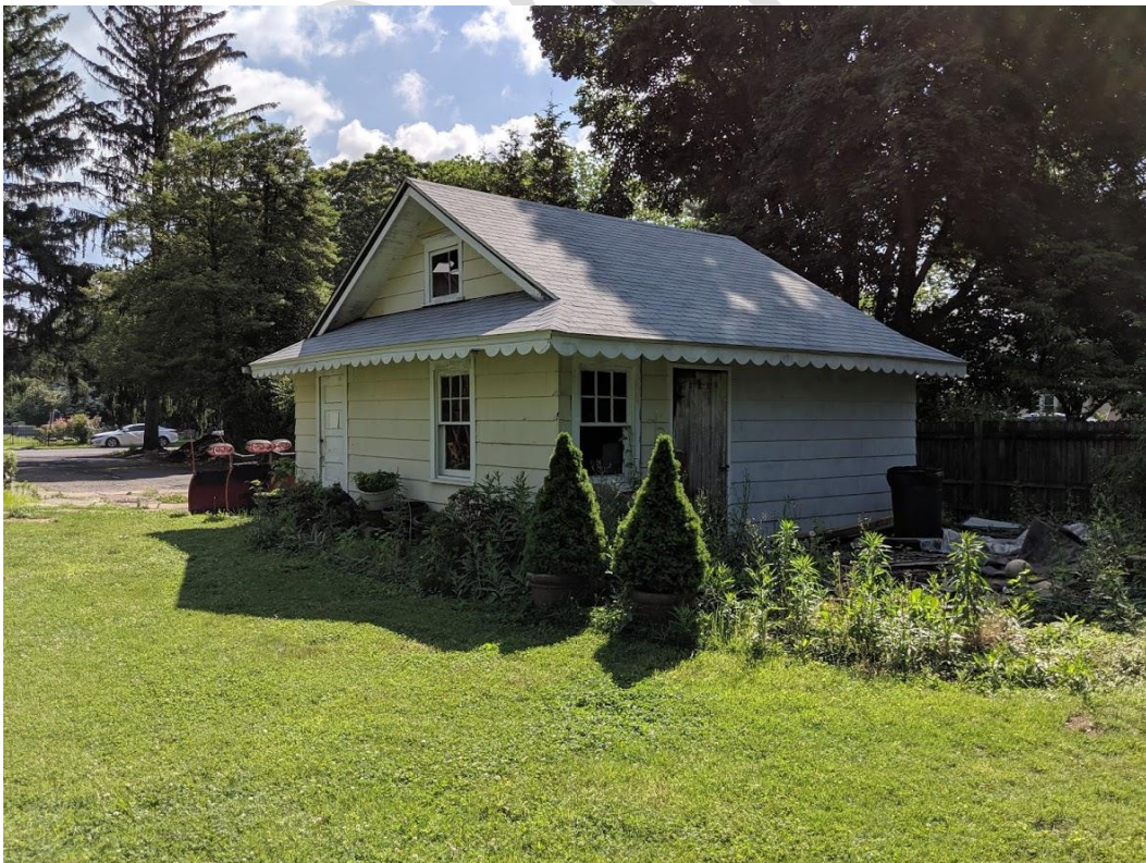
Photograph 45: Block 39 Lot 7 Garage (Rear)
