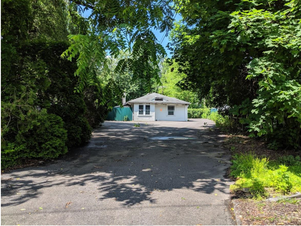
Photograph 36: Block 39 Lot 5 Front Facade of Building, from Washington Road
