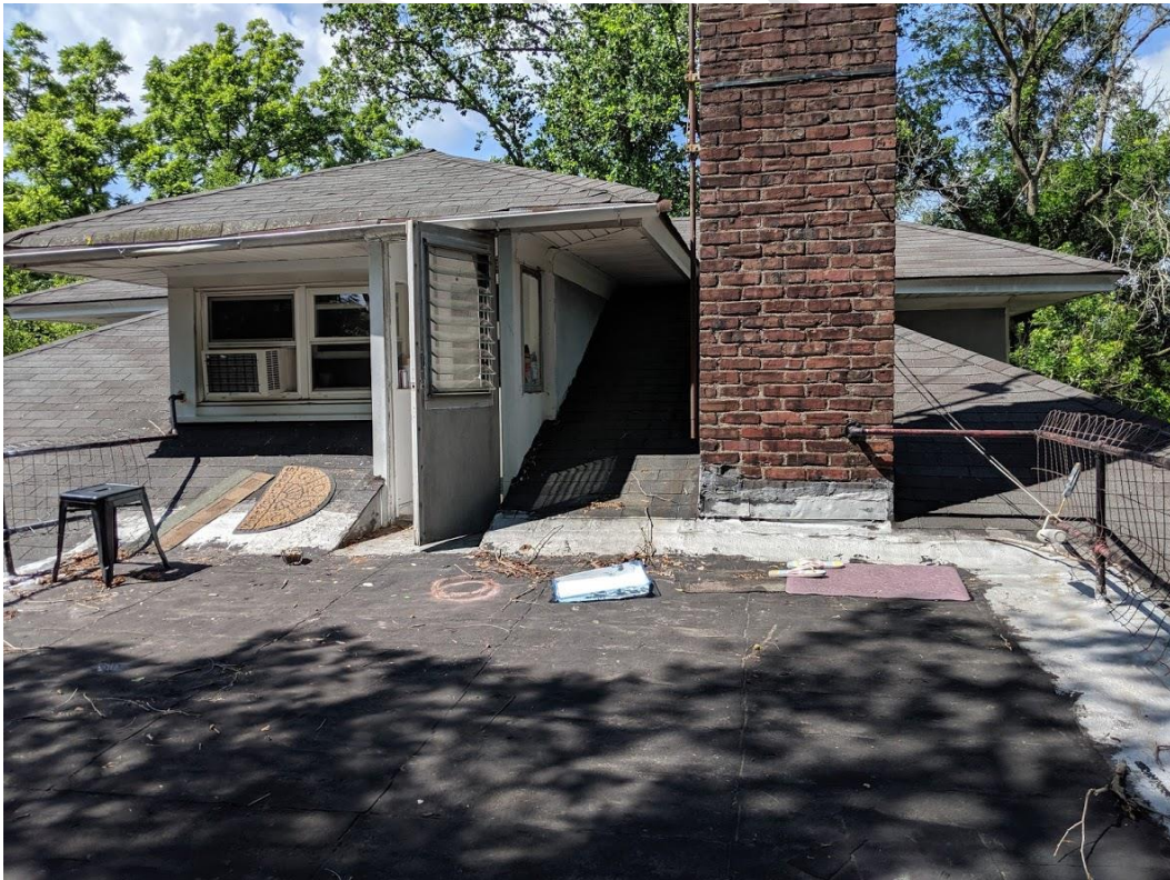
Photograph 29: Block 39 Lot 4 Roof above Northeastly Side Façade of Building
