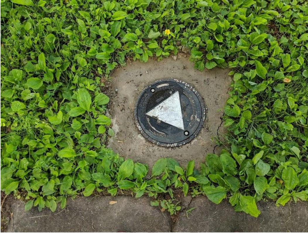
Photograph 34: Block 39 Lot 4 Monitoring Well
