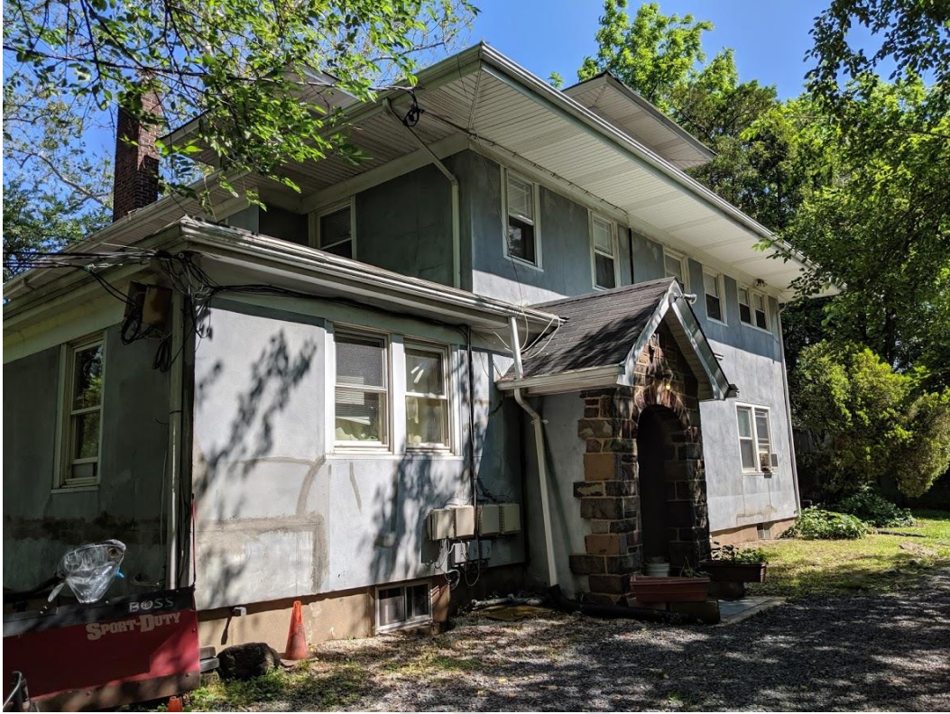
Photograph 26: Block 39 Lot 4 Rear Façade of Building
