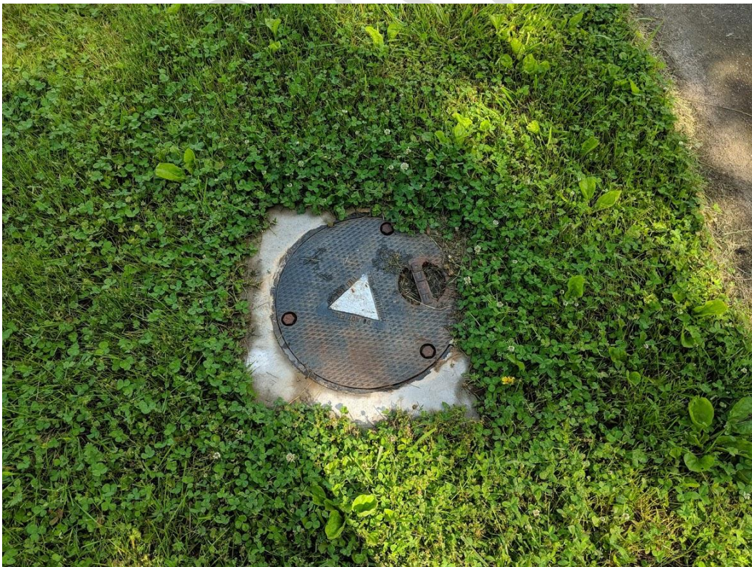
Photograph 33: Block 39 Lot 4 Monitoring Well
