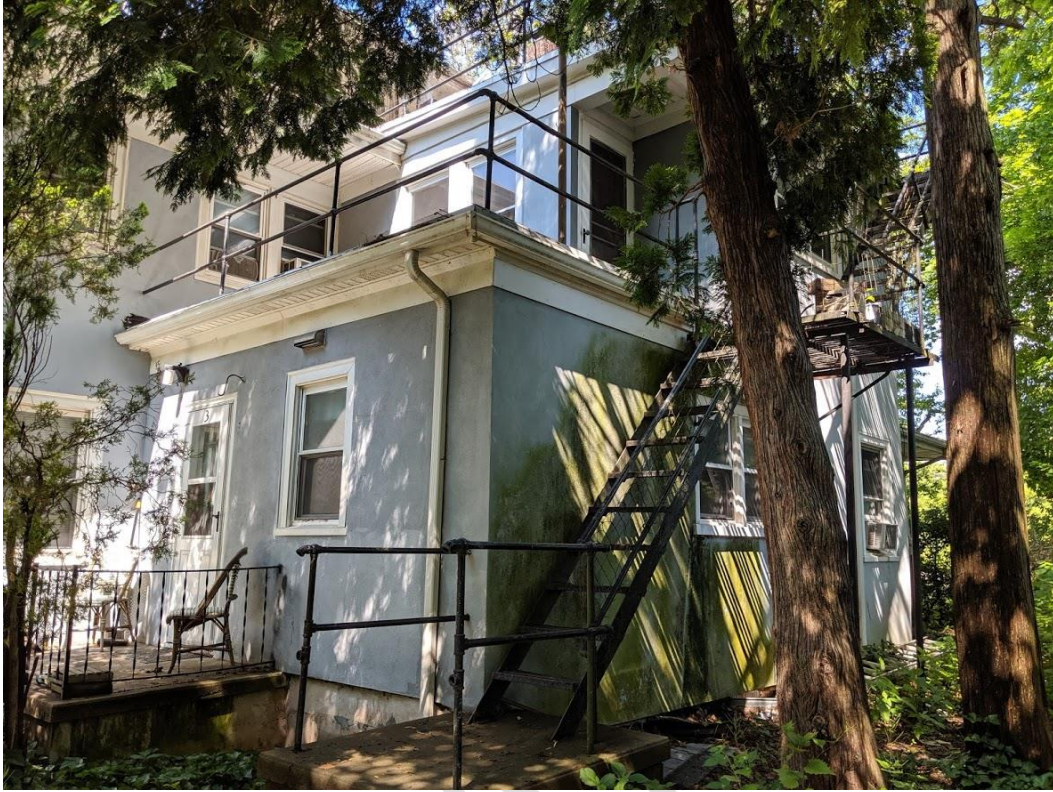
Photograph 28: Block 39 Lot 4 Northeastly Side Façade of Building
