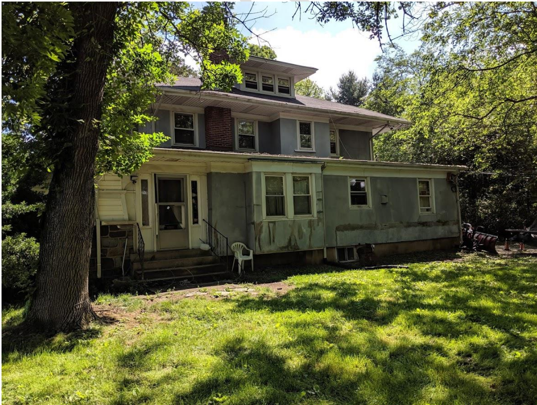
Photograph 23: Block 39 Lot 4 Southwesterly Side Façade of Building
