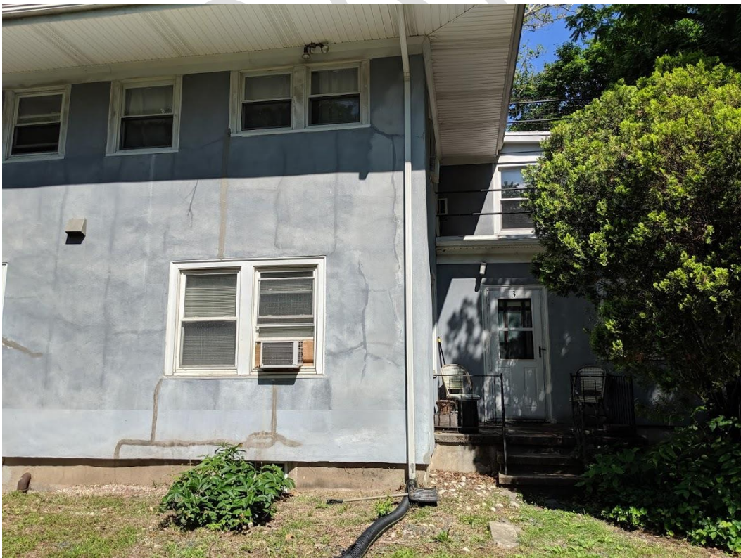
Photograph 27: Block 39 Lot 4 Rear Façade of Building
