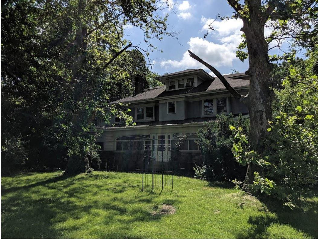
Photograph 22: Block 39 Lot 4 Front Façade of Building
