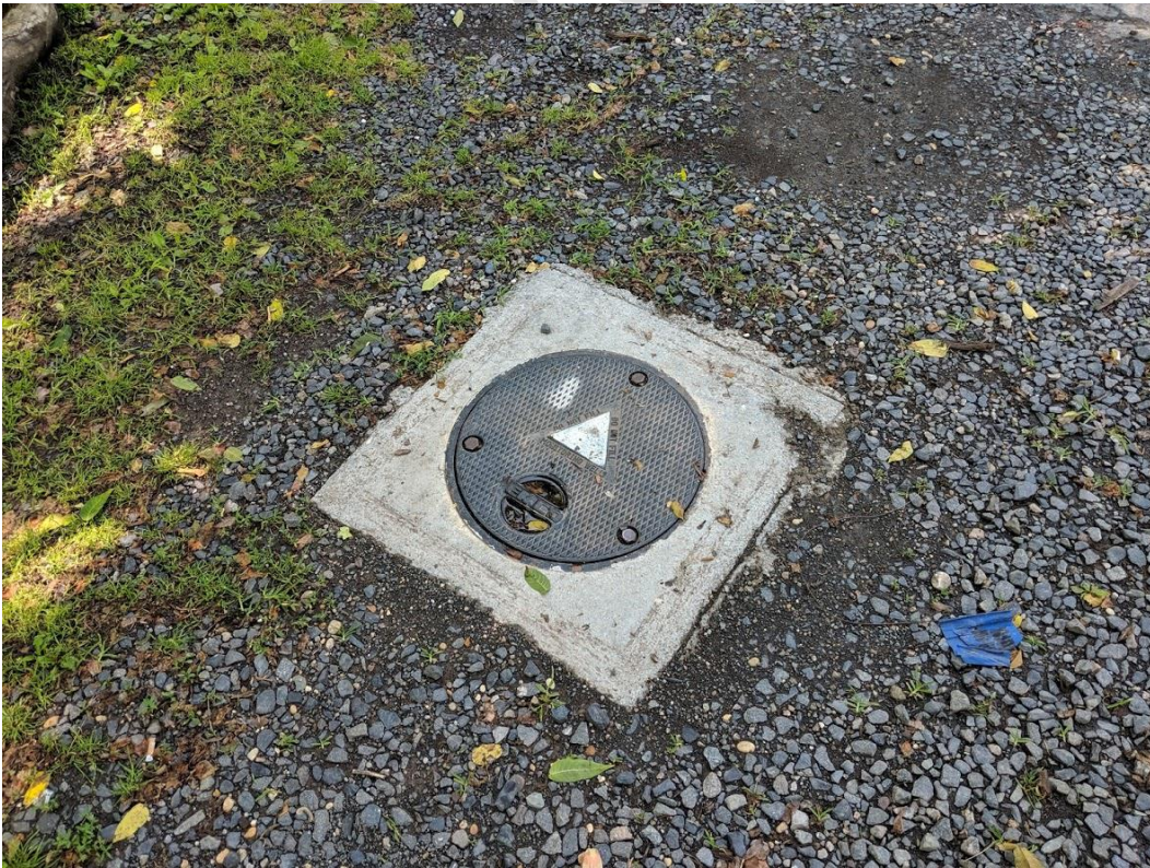
Photograph 35: Block 39 Lot 4 Monitoring Well
