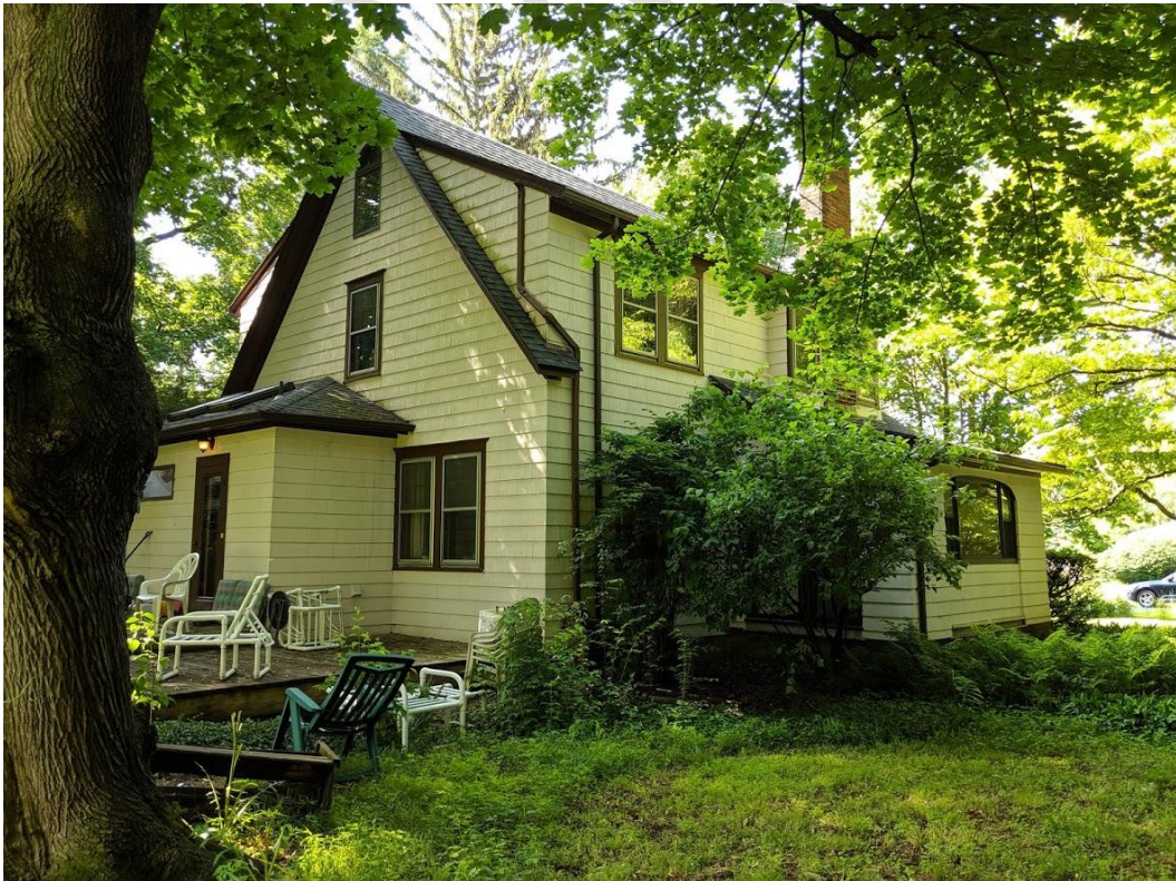
Photograph 50: Northerly Side Facade of Dwelling
