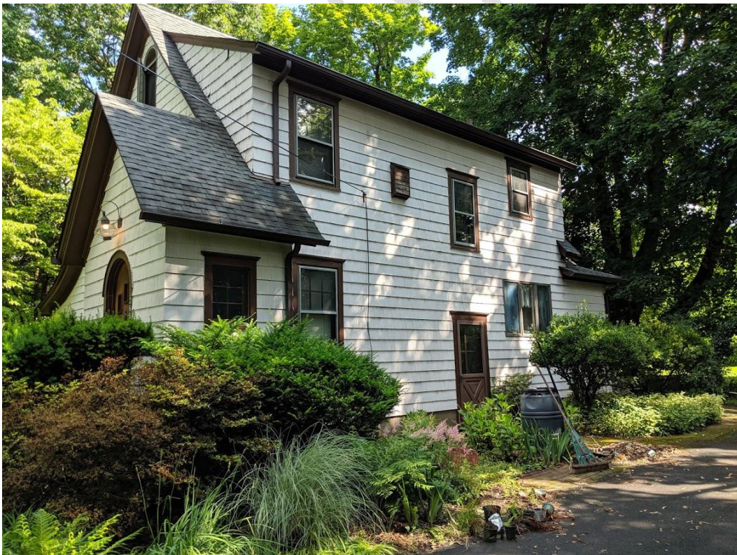
Photograph 48: Southerly Side Façade of Dwelling
