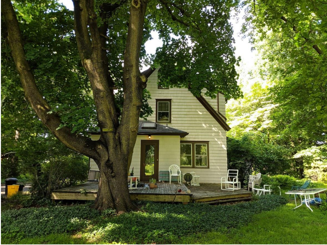
Photograph 49: Rear Façade of Dwelling
