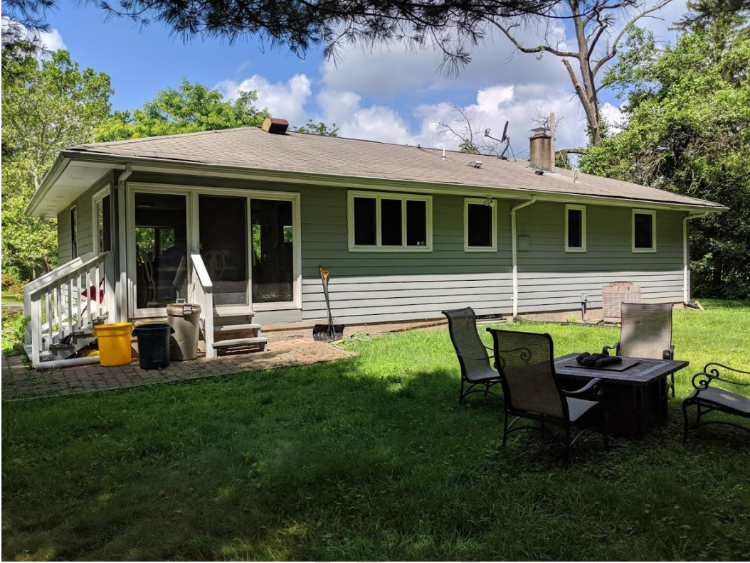
Photograph 20: Block 38 Lot 45 Rear Facade of Dwelling
