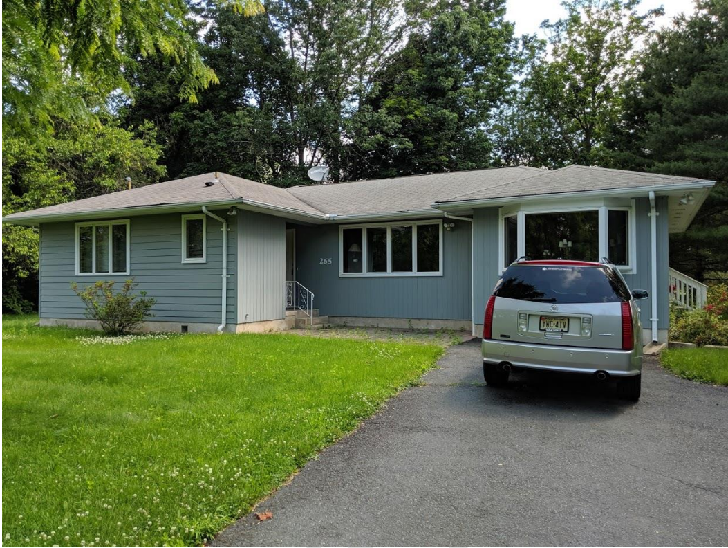
Photograph 18: Block 38 Lot 45 Front Facade of Dwelling
