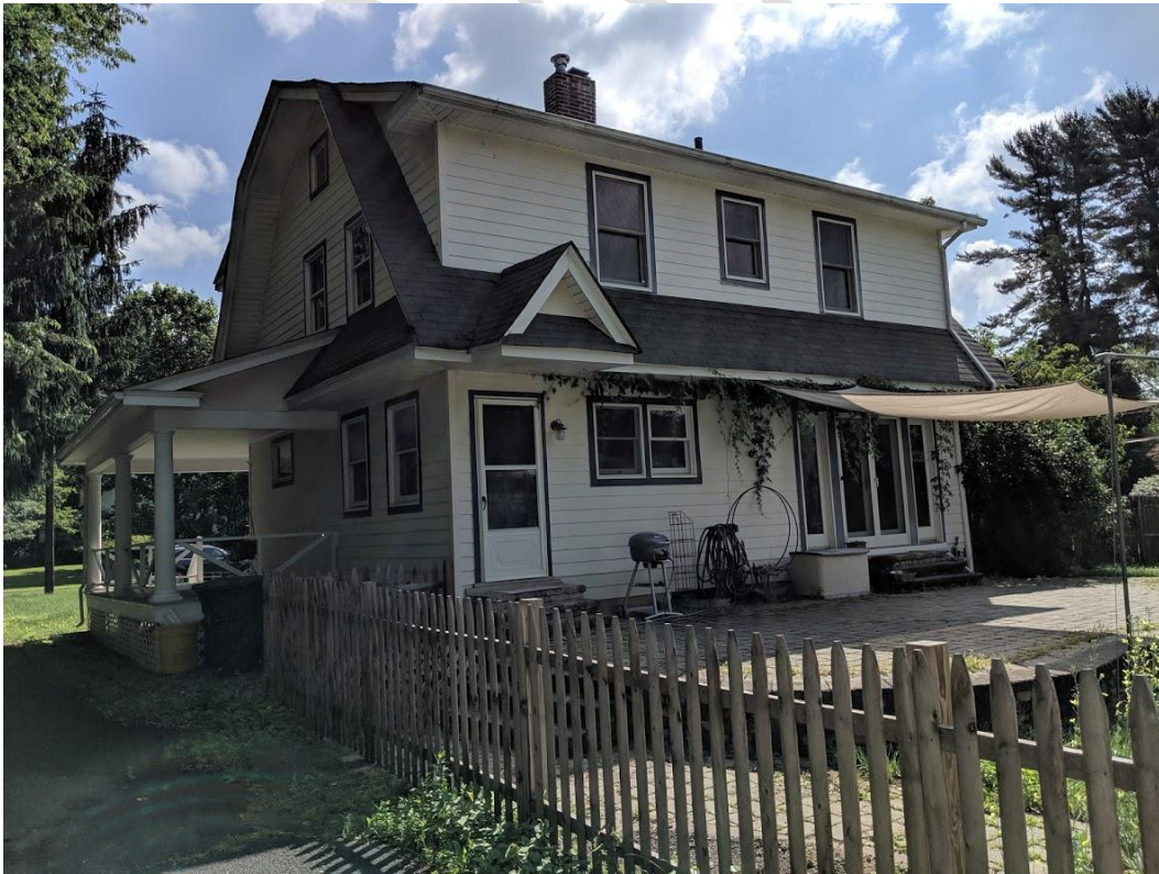
Photograph 17: Block 38 Lot 25 Rear Façade of Dwelling
