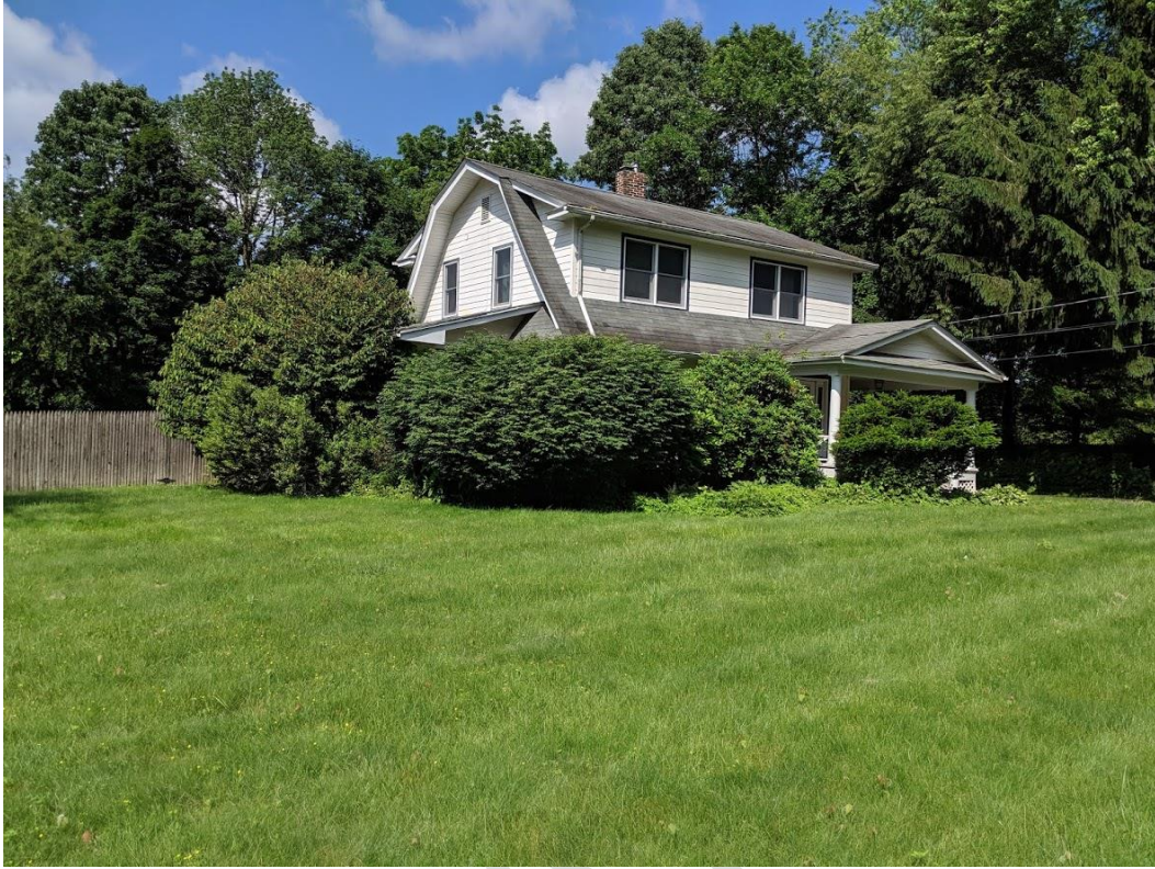
Photograph 14: Block 38 Lot 25 Easterly Corner, Looking Southwest
