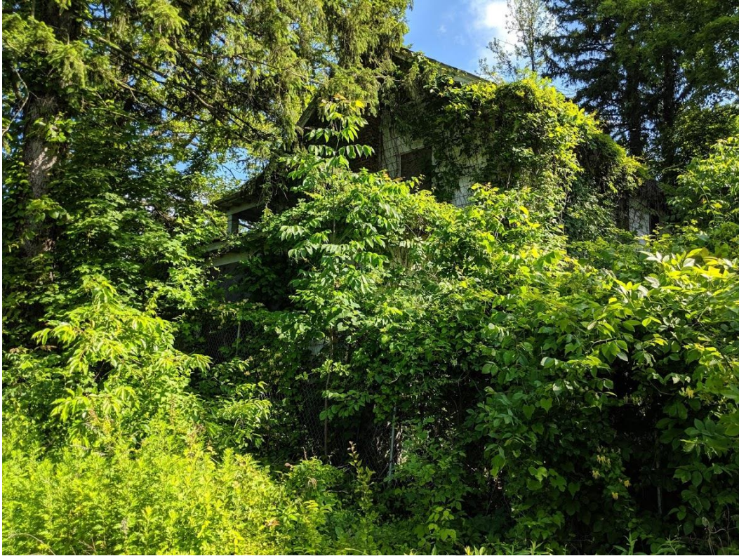
Photograph 5: Block 38 Lot 2 Westerly Side Facade of Dwelling
