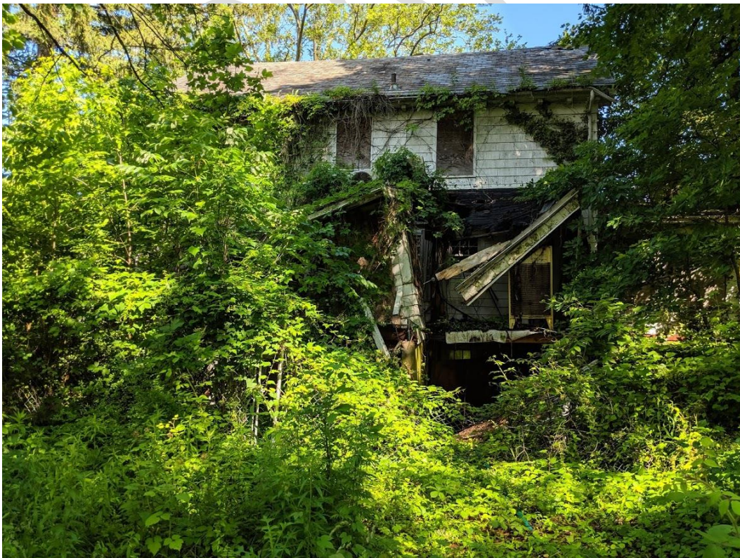
Photograph 6: Block 38 Lot 2 Rear Facade of Dwelling
