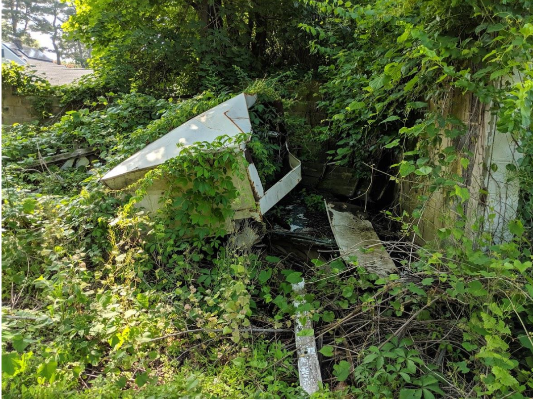
Photograph 9: Block 38 Lot 2 Rear Yard
