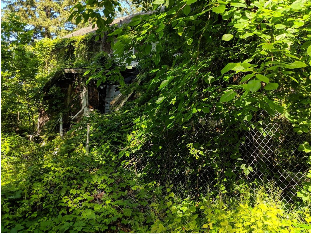
Photograph 7: Block 38 Lot 2 Rear Facade of Dwelling
