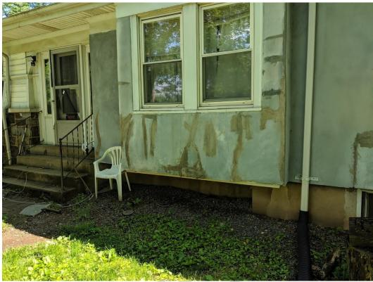
Photograph 24: Block 39 Lot 4 Southwesterly Side Façade of Building (showing patchwork of cracks)
