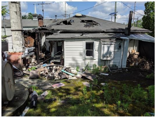
Photograph 37: Block 39 Lot 5 Southerly Side Façade, Showing Fire Damage (photo taken from Lot 7)
