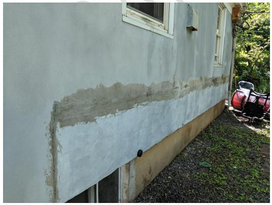
Photograph 25: Block 39 Lot 4 Southwesterly Side Façade of Building (showing patchwork of cracks)
