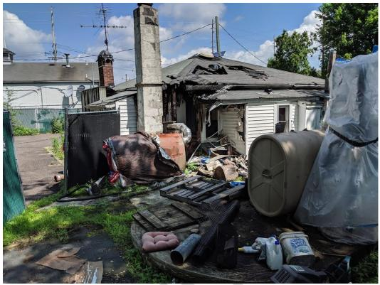
Photograph 38: Block 39 Lot 5 Southerly Side Façade, Showing Fire Damage (photo taken from Lot 7)
