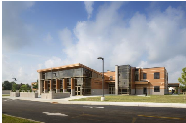
Village School Addition - Completed
