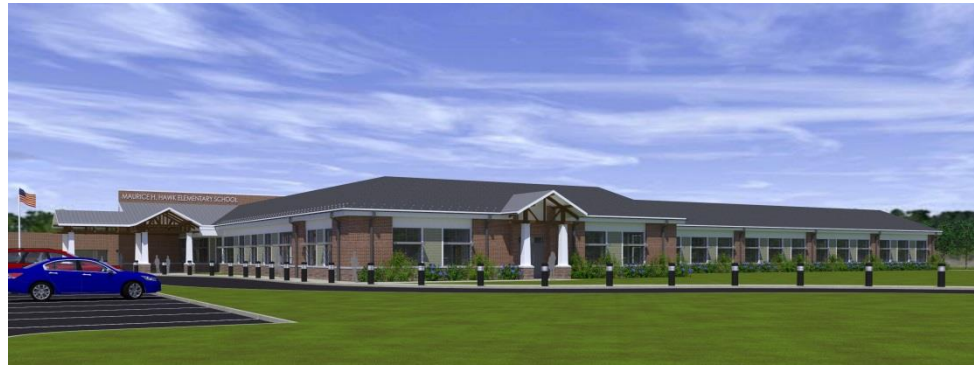
Maurice Hawk School Addition - Summer 2018
